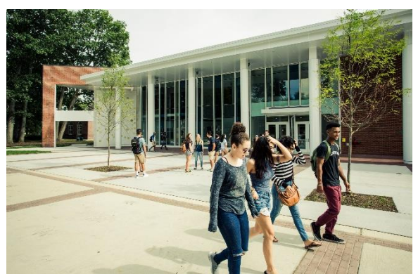
FIGURE 43 - EXTERIOR VIEW OF THE BROWER STUDENT CENTER
