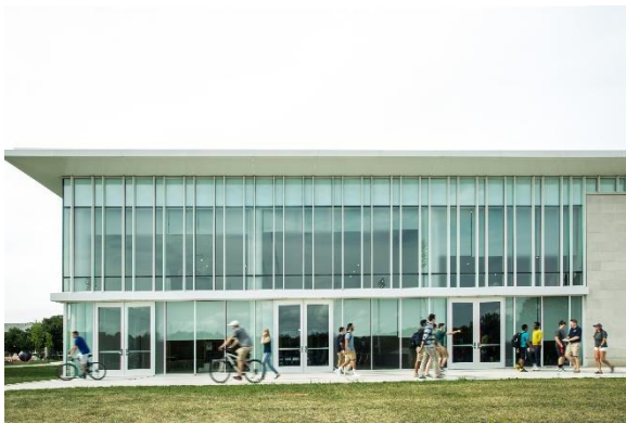
FIGURE 46 - EXTERIOR VIEW OF THE BROWER STUDENT CENTER
